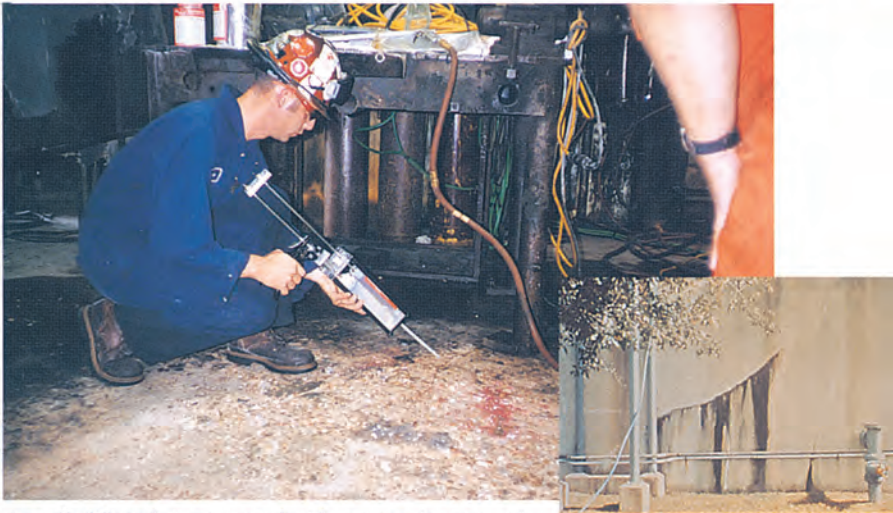
A spalled floor being injected with epoxy prior to repair.
