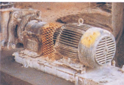
Same pump base repaired
