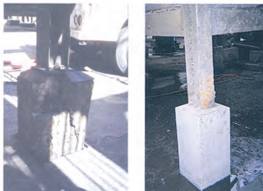
Spalled, cracked pedestal (left) is fully restored (right).
