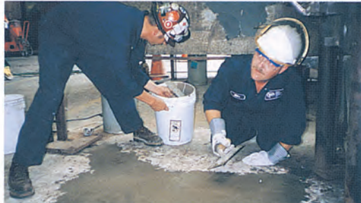
Badly spalled floor area being prepared with a high strength repair material.
