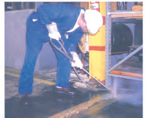
A Team technician (above) cleans an EVA expansion joint prior to repair. Below, Team technicians complete repairs on the same expansion joint.
