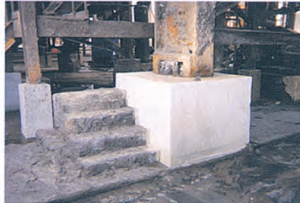
Same pedestal restored and strengthened
