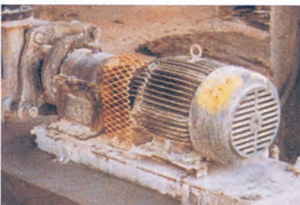
Same pump base repaired
