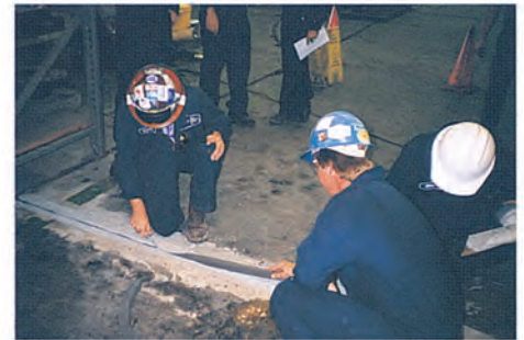
A Team technician (above) cleans an EVA expansion joint prior to repair. Below, Team technicians complete repairs on the same expansion joint.
