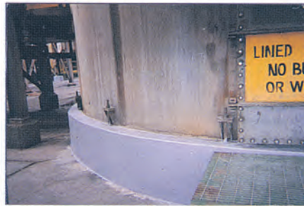
Same tank base repaired and strengthened
