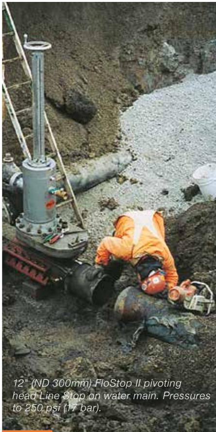
12" (ND 300mm) FloStop II pivoting head Line Stop on water main. Pressures to 250 psi (17 bar).
