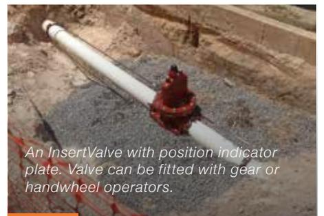
*An InsertValve with position indicator plate. Valve can be fitted with gear or handwheel operators.*
