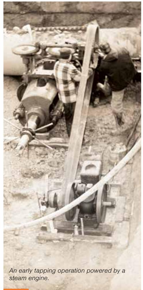
*An early tapping operation powered by a steam engine.*
