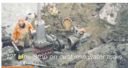
12" Line Stop on cast iron water main
