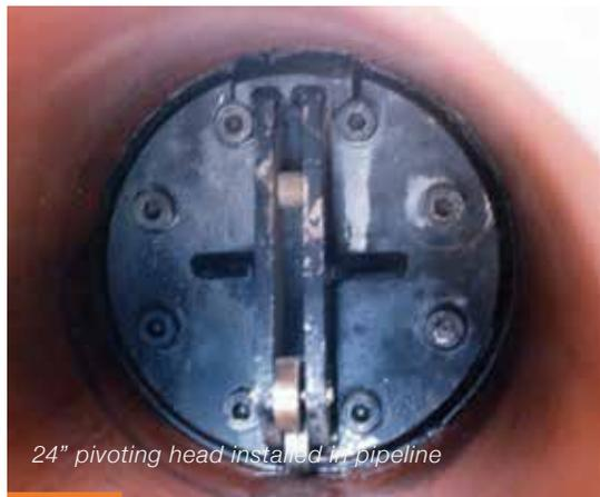
24" pivoting head installed in pipeline
