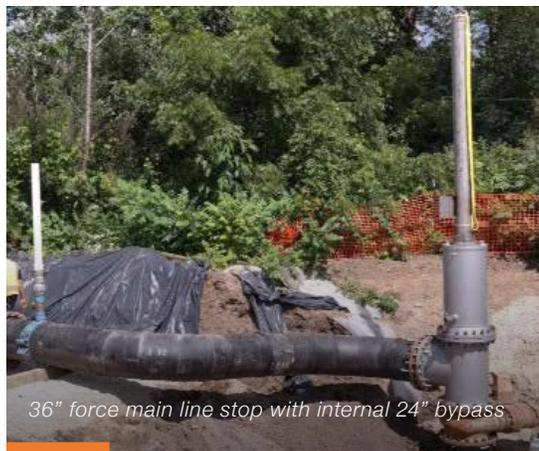
36" force main line stop with internal 24" bypass
