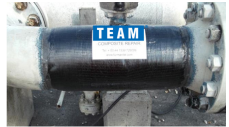
TEAM Advanced Carbon Fiber Composite Repair at Touch Point
