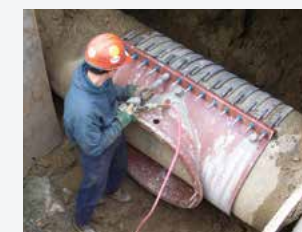
Sleeve grouted and tightened around pipe
