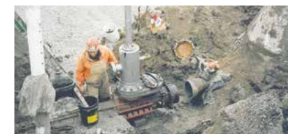
12" Line Stop on cast iron water main
