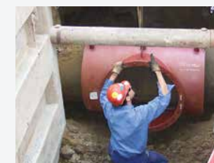
Concrete tapping sleeve mounted
