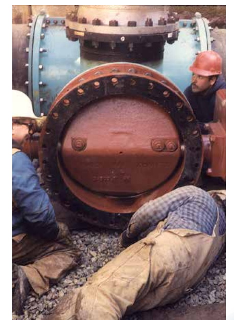
CUSTOM APPLICATIONS Like this installation of 24" butterfly valve during tapping operation.
