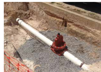
An InsertValve with position indicator plate. Valve can be fitted with gear or handwheel operators.
