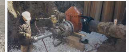
16"x16" Tap on cast-iron pipe
