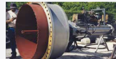
60" Hot / Wet Tap preparation
