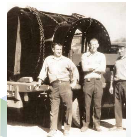
An original tapping crew prepares for a 48" tap.
