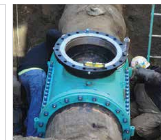
Mechanical joint line-stop fitting installation
