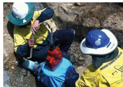
An InsertValve installation under full line pressure.
