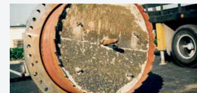
48" concrete Hot / Wet Tap coupon
