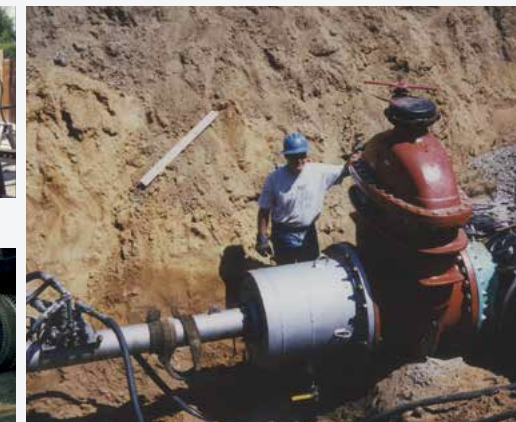
30" Hot / Wet Tap on ductile iron pipe
