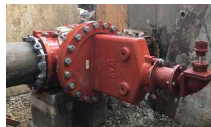
The InsertValve can be installed in any orientation on any type of pipe material.
