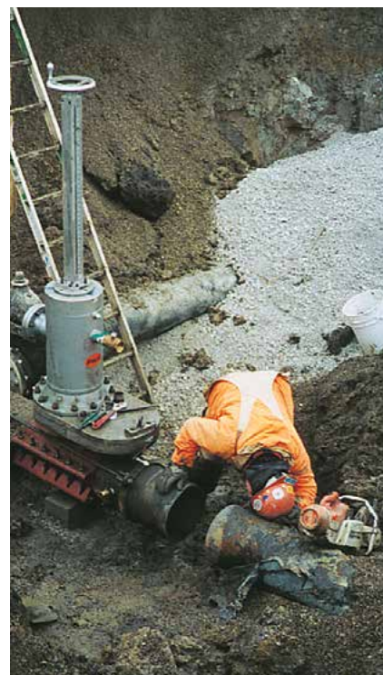
12" (ND 300mm) FloStop II pivoting head Line Stop on water main. Pressures to 250 psi (17 bar).
