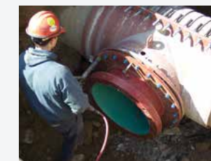
Gland installed and sleeve pressure-tested
