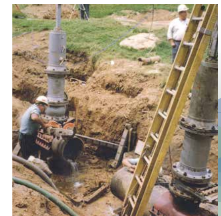
24" Line Stops (valve cut in)
