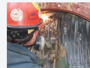
Cutting torch removes reinforcing steel wires
