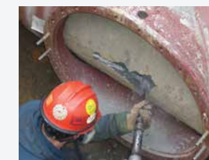
Chipping gun removes mortar coating
