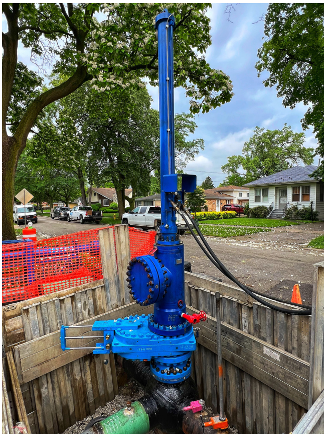
Figure 2. SmartStop deployed through a spherical fitting.
